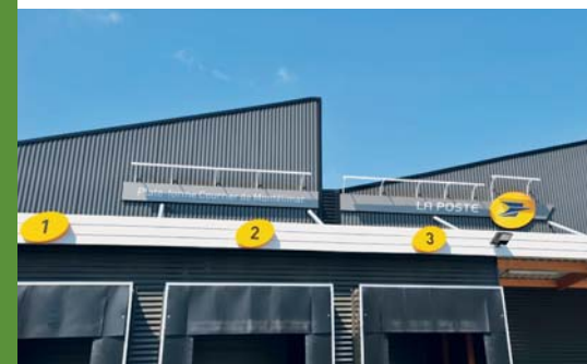
The Montélimar Mail hub, inaugurated in 2009, is the first postal building that meets the HEQ standard "NF Bâtiments tertiaires" for service-sector buildings.
